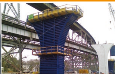
HUEY P. LONG BRIDGE Jefferson Parish, Louisiana
