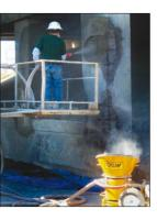
machine conveys materials up to 1000 ft. horizontally and 300 ft. vertically. Applications include drainage ditches, tunnels, retaining walls, pools, and rockscapes. Gunite Supply & Equipment. 888-321-5526. www. gunitesupply.com.
