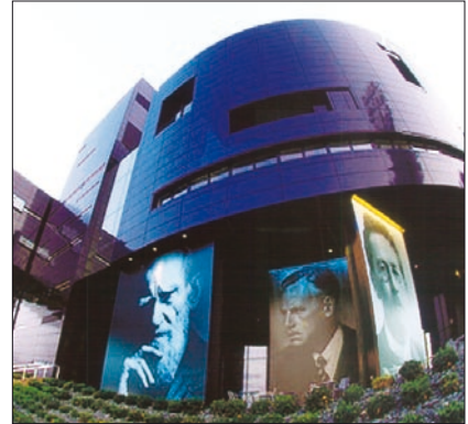
Honored as this year's PTI Project of the Year, Award of Excellence, the New Guthrie Theater Center in Minneapolis integrated post-tensioned concrete into a uniquely designed building. Photo: PTI
