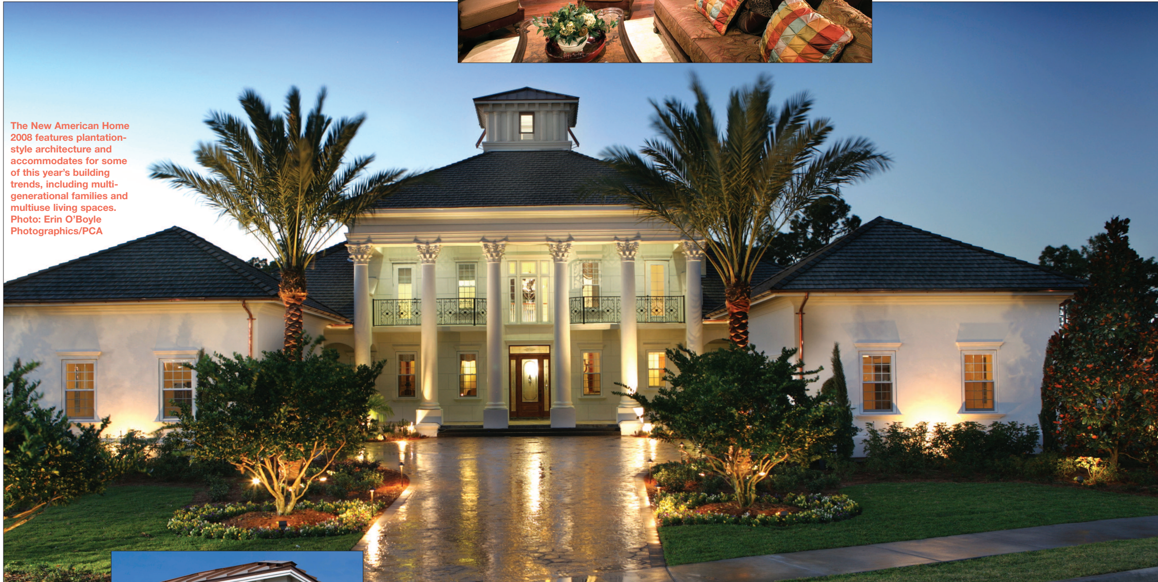
Left: Concrete roof tiles were finished with a cement-based stucco system and completed cupola—a traditional element found in Victorian architecture. Photo: Erin O'Boyle Photographics/PCA
