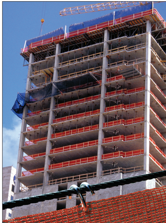
This shows both a vertical guardrail netting and a perimeter netting system in place on a commercial building construction site. Photo: Capital Safety
